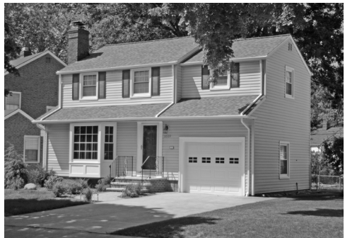
Edison Road home after renovation
