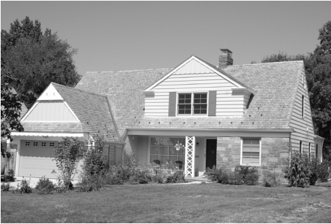
Westover Road home after renovation
