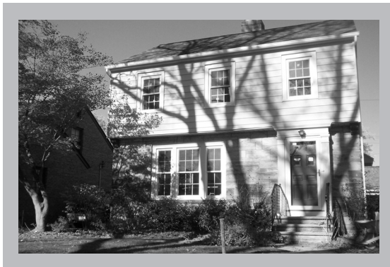
Berkeley Road home after renovation
