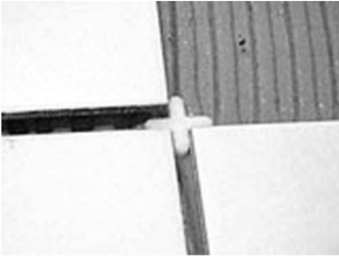
Spacers keep grout width consistent
