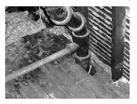
Check for holes that may have been drilled for wiring, and use caulk or spray foam to close them. Chimneys should not have any combustibles against them and may require metal flashing and high heat caulk to seal air leaks. It is especially important to duct exhaust fans and clothes dryers to the outside to reduce humidity in the attic.
