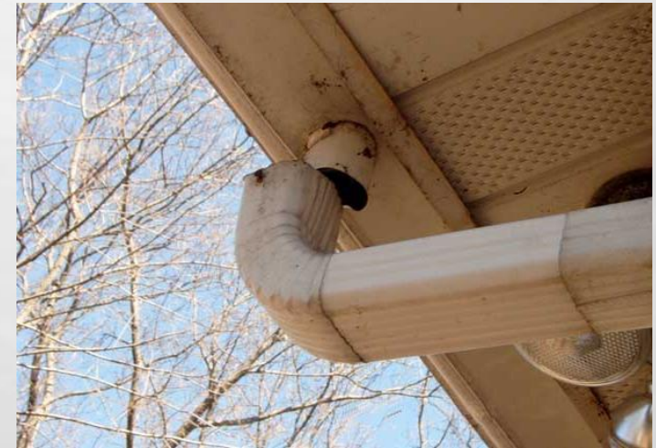
BROKEN DOWNSPOUT
