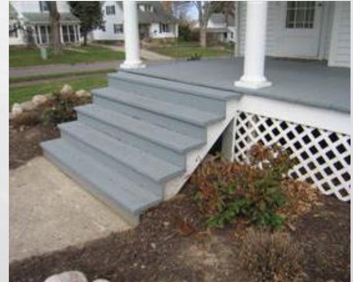
MISSING HANDRAILS
