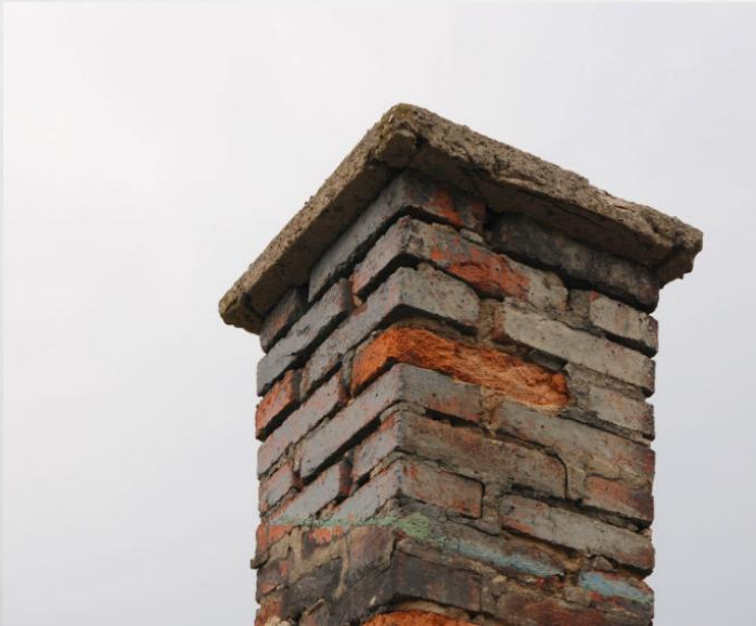
MISSING MORTAR
