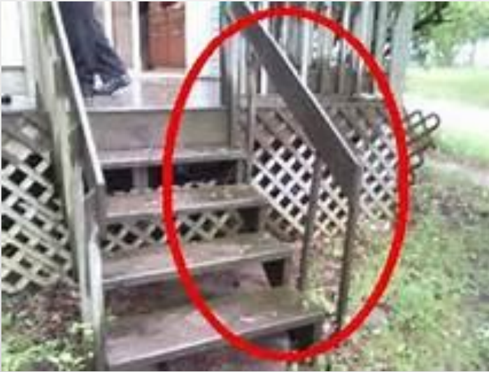
BROKEN HANDRAILS
