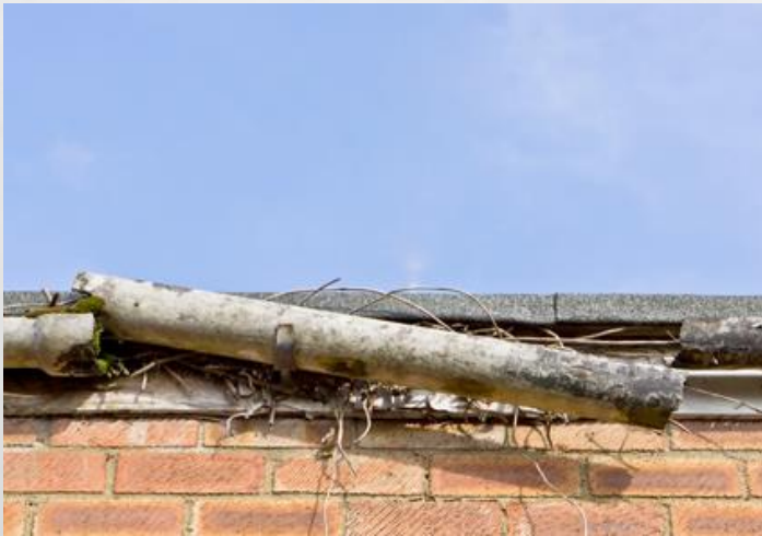
BROKEN GUTTER
