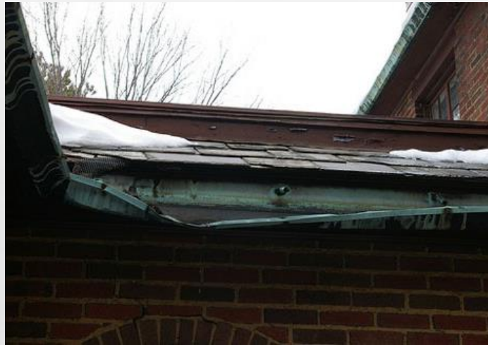
DAMAGED GUTTER
