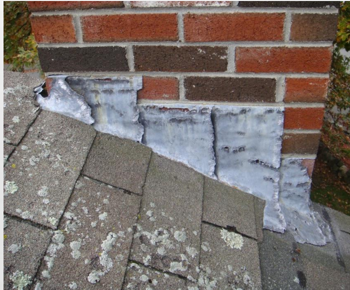
DAMAGED FLASHING
